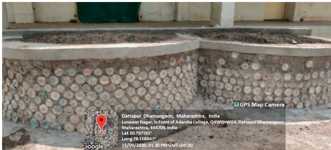
Eco-Bricks Installed at Commerce Department
