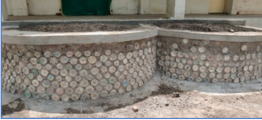
Construction work for Eco Bricks prepared From Single use plastic
