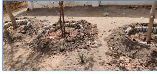
Construction work for Eco Bricks prepared From Single use plastic
