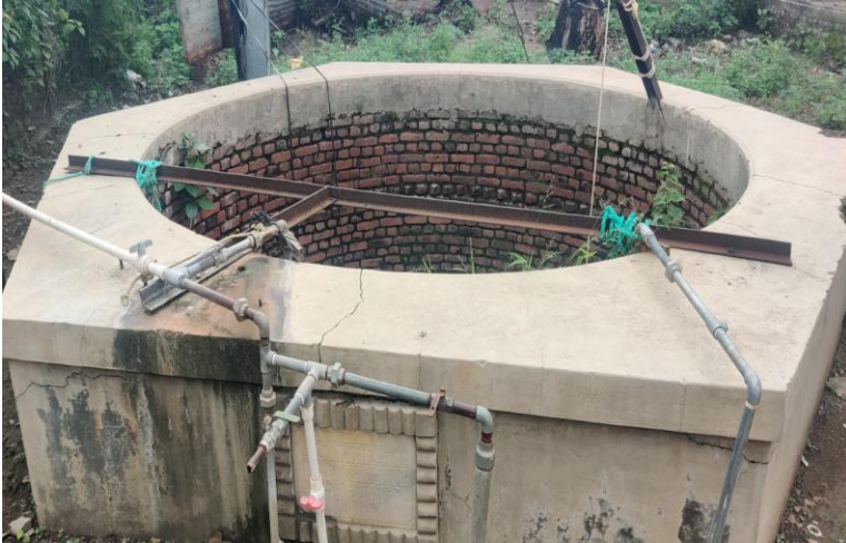
WATER WELL WITH PIPE
